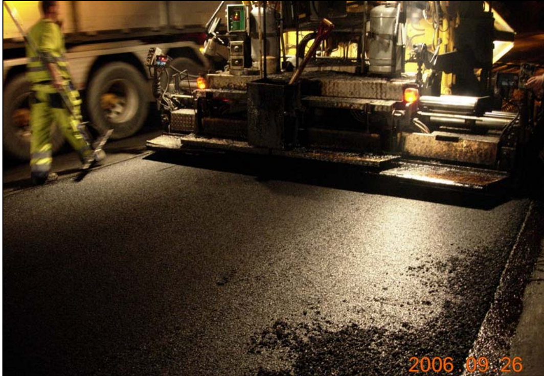
Figure 7. Installment of the poroelastic asphalt pavement.
